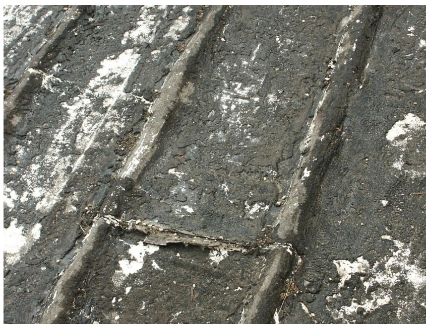
Detail of damages on the roof of the Church of the Nativity
